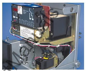
A. Feed the Sensor Harness through the grommet in the left side of the Aux. CT Module. Connect the Sensor Harness to the proper terminals of the Aux. CT Module. Refer to Section 12 of the Retrofit Application Data, supplied with the Retrofit Kit, for detailed wiring specifications.
