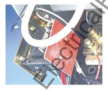
NOTE: The power convention of the DB-25 Breaker is normally Top to Bottom, meaning the Top Breaker Stabs are on the Line Side of the Breaker and the Bottom Breaker Stabs are on the Load Side.
