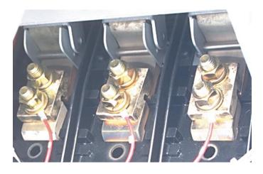
A. Route the PT Wires between the left Trip Unit Assembly Mounting Bracket and the left Arc Chute. Continue by routing the PT Wires down into the Breaker towards the Copper Connectors installed in Step 3.
