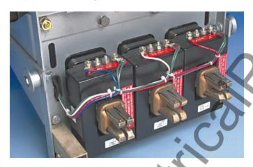
A. Slide a Sensor over each bottom Breaker Stab. The terminals of the Sensors should face upwards.
