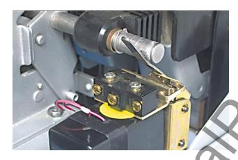
G. Mount the DTA Assembly to the right side of the Breaker Platform using the DTA Mounting Clip, (1) .190-32 x .750" screw, (2) flat washers, (1) lock washer, and (1) nut, and the (1) .250-20 x .500" Sems screw and (1) flat washer provided.
