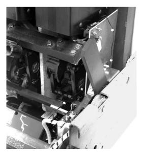
H. For Kits Supplied with a Breaker Mounted CPT Only. Route the Line Side HV Wires along the right rear side of the Breaker to the bolts below the top Breaker Stabs.
