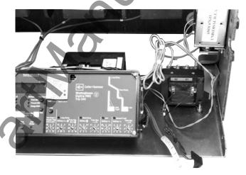
E. Attach the Glass Poly Insulation Plate to the top of the CPT, as shown, using the screws and lock washers supplied with the CPT kit.
