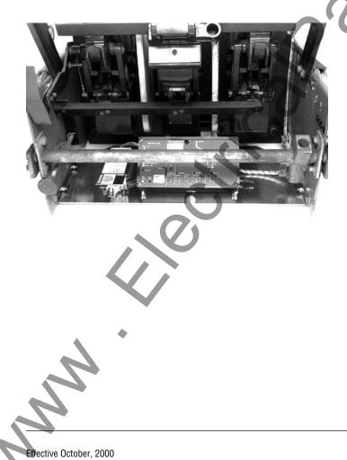
F. Route the External Harness towards the right side of the Breaker, then up towards the DTA Assembly. Remove the top front screw securing the DTA mounting bracket. Using the two wire clamps and the screws provided, secure the External Harness to the DTA.
