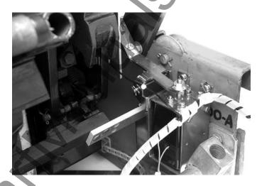
G For Kits Supplied With An Auxiliary Switch Only. Route the two wires, with ring terminals, from the External Harness along the right side of the Breaker to the Microswitch Switch. Connect one wire to the normally "Open" terminal and the other wire to the "Common" terminal.
