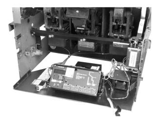
A. Align the holes in the Breaker Mounted CPT with the predrilled holes in the Trip Unit Mounting Platform, as shown, then secure using the (4) .190-32 × .500" screws, (8) flat washers, (4) lock washers, and (4) nuts supplied. Note that the mounting screws must be inserted from the bottom of the Mounting Platform and that the X1 and X2 terminals must face the front of the Mounting Platform.
