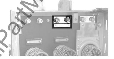
C. Remove and discard the six bolts and washers (one row) located directly below each top Finger Cluster.
