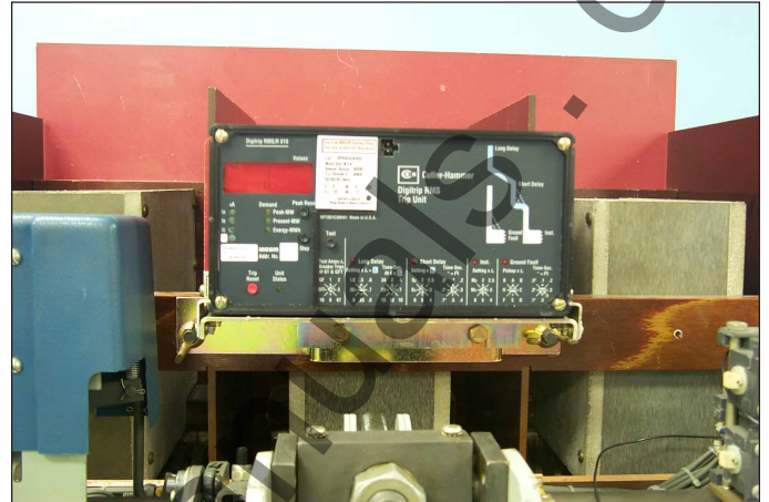
Fig. 48 Overview: Trip Unit Installed on the Breaker.
