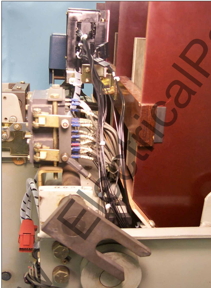
Fig. 59 External Harness Connections at the Trip Unit.
