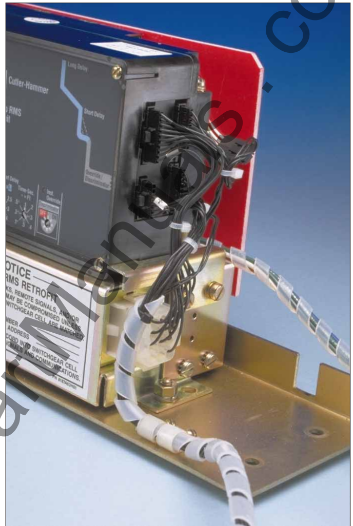
Fig. 9 External Harness connected to the Trip Unit.
