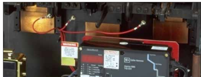
Fig. 18 PT Wires connected to the Phase Frames.
