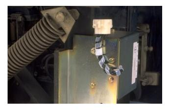
E. Connect the Sensor Harness to the proper terminals on the Aux. CT Module. Refer to Section 12 of the Retrofit Application Data, supplied with the Retrofit Kit, for detailed wiring specifications.
