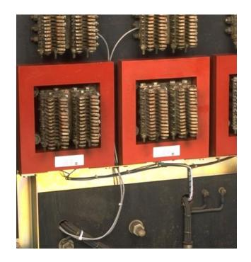
C. Cut the HV Wires to the appropriate length for attachment to the appropriate top Breaker Stabs. Strip .250" from each HV Wire and attach a .250" ring terminal.
