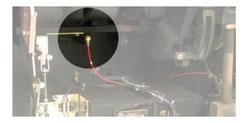
Use the wire clamp provided and the existing screw to secure the PT Wires to the top of the Aux. CT Module.
