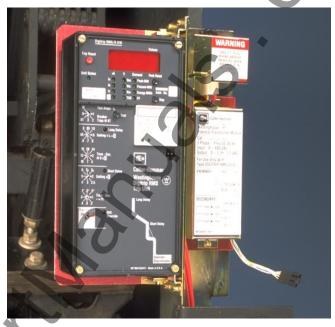
. While holding the Breaker Control Panel in place, remove the two (2) copper bolts, washers and nuts that secure the Control Panel Assembly to the Breaker Control Panel Assembly Mounting Bracket.
