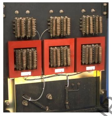
Note: The power convention of the ITE LG-3000 (Frameless) Breaker is normally *Top to Bottom*, meaning the Top Breaker Phase Frames are on the *Line Side* of the Breaker and the Bottom Breaker Stabs are on the *Load Side*.
