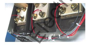
P. Attach the appropriate label for the Breaker in a clearly visible position. Three (3) labels are included with the CPT, one (1) for 480 Volt, one (1) for 240 Volt, and one (1) for 208 Volt systems.
