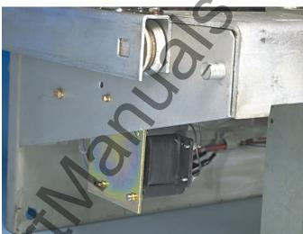
A. Temporarily align the CPT Mounting Bracket with the existing holes in the left Breaker Frame, as shown.
