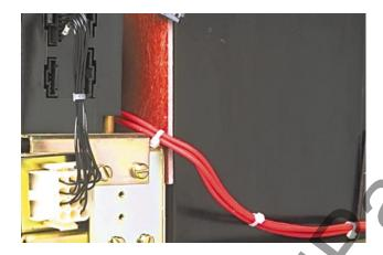
Step 7: Connecting Sensor Harness and DTA Wires to the Aux. CT Module
