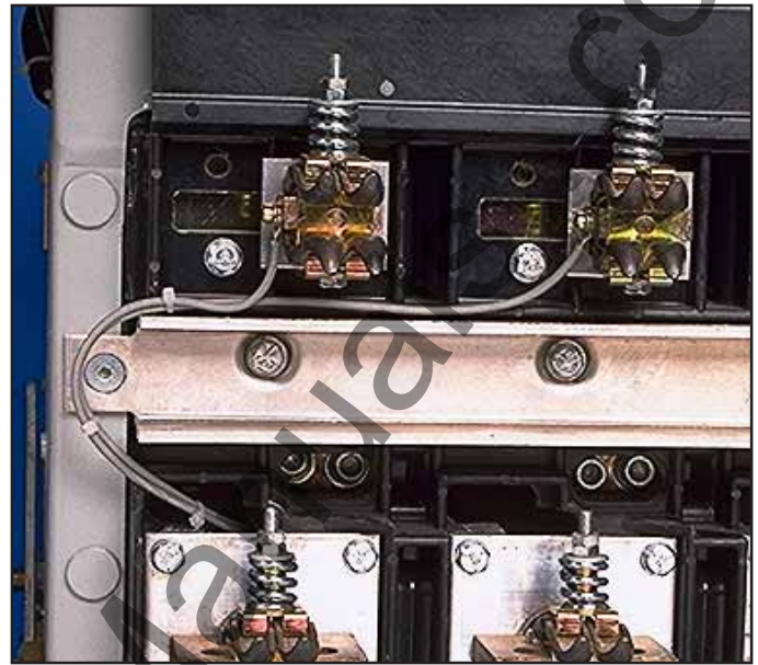
Fig. 14 Routing of the HV Line Side Wires.
