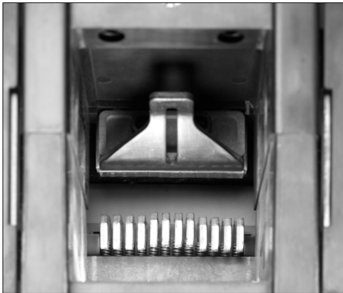
Figure 6-3 Primary Contacts with Circuit Breaker Open (Not Used for Contact Wear Inspection)
