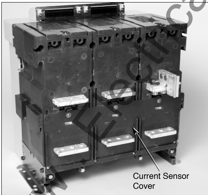
Figure 6-7 Current Sensor Cover in Place Over Sensors
