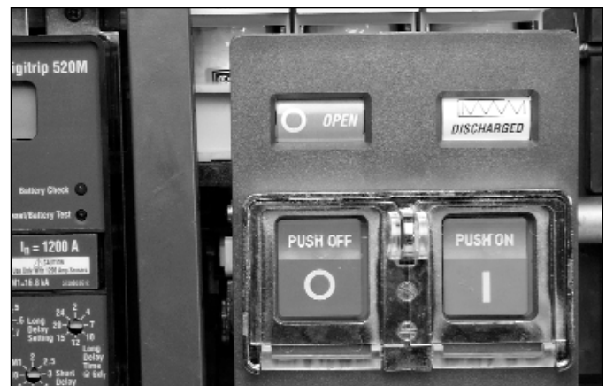
Figure 3-59 ON-OFF Pushbutton Lockable Cover Plate
