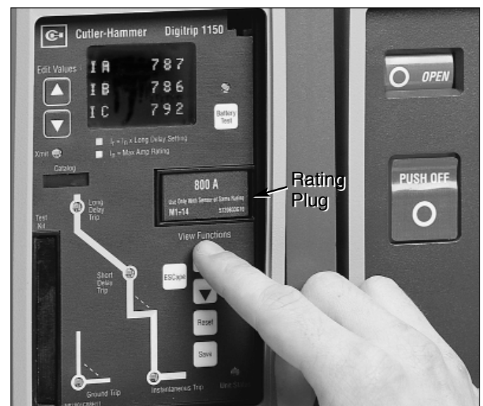
Figure 6-6 Trip Unit Rating Plug Location
