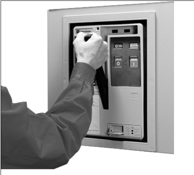
Figure 3-12 Circuit Breaker Closing Springs Being Manually Charged
