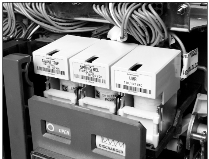
Figure 3-52 Shunt Trip, Spring Release and Undervoltage Release Installed
