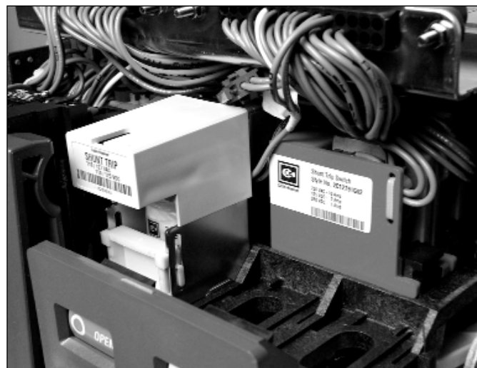
Figure 3-49 Shunt Trip Switch Installed
