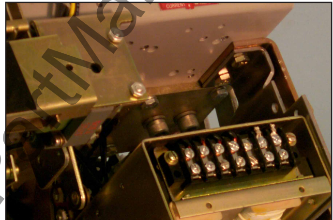
Fig. 8 Aux. CT Module Installed in the Breaker.
