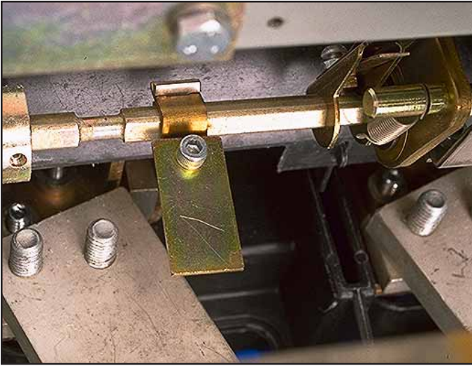
Fig. 12 Trip Finger Extension Plate Installed on the Trip Finger.
