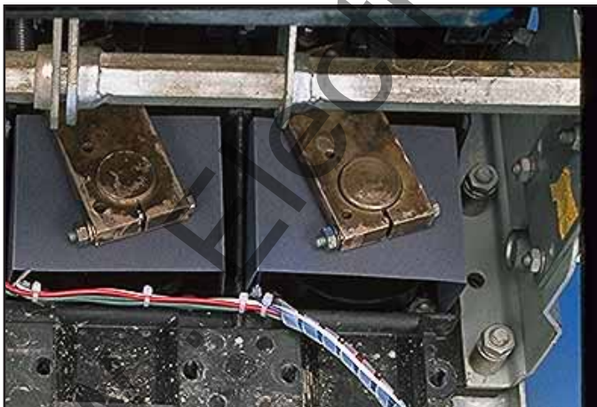
Fig. 4 Shields Installed Over the Sensors.
