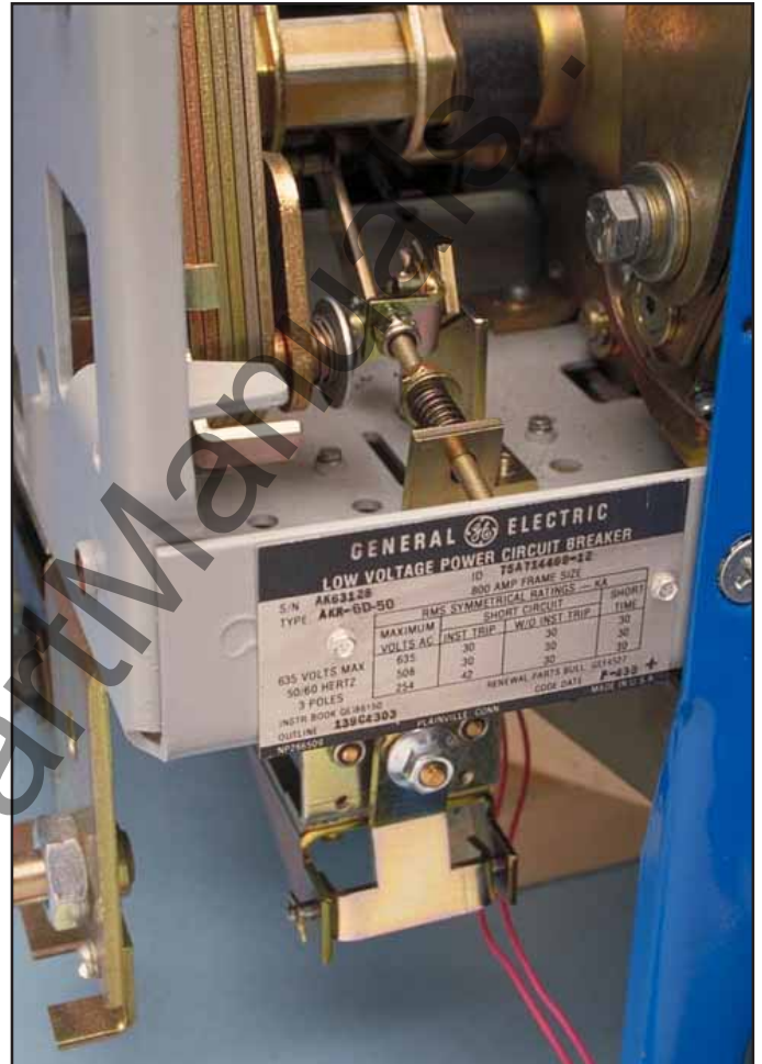
Fig. 11 DTA and Reset Assemblies Installed in the Breaker
