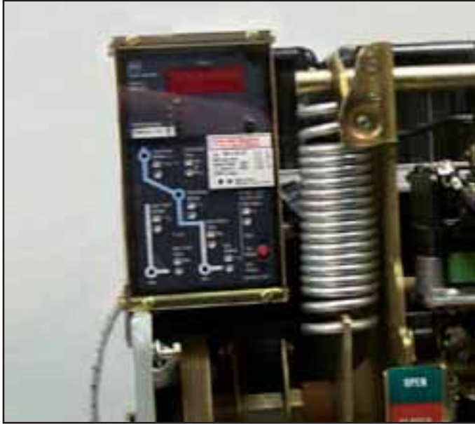
Fig. 22 Overview: Trip Unit Installed on the Breaker.
