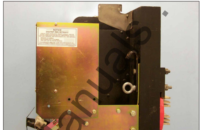
Fig. 32 Digitrip Nameplate Installed on the Breaker.
