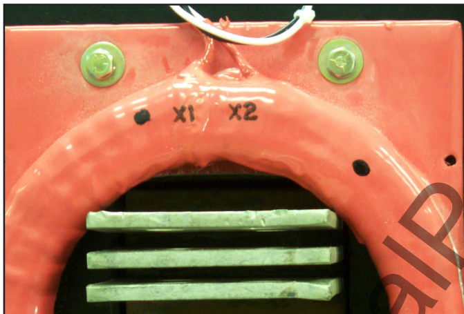
Fig. 3 Correct Positioning of the "X" Markings for the Phase 1 and 3 Top Sensors.
