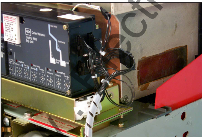
Fig. 62 External Harness Connections at the Trip Unit.
