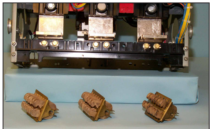
Fig. 5 Finger Clusters Removed from the Bottom Load Terminals (Electrically Operated).
