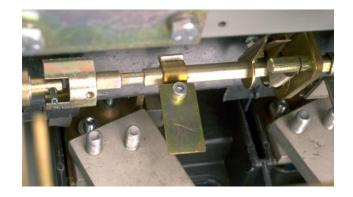
B. Align the Reset Pivot Assembly with the existing holes in the Breaker Shelf. Apply Loc-Tite® 242 to the threads then mount the Reset Pivot Assembly using the (2) .164-32 × .375" screws, (2) lock washers, and (2) flat washers supplied.
