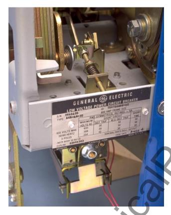
G. Adjust the DTA Gap Adjustment Screw to achieve a gap between the screw head and the Trip Finger of approximately .09" to .12".
