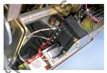
NOTE: The power convention of Circuit Breakers is normally Top to Bottom, meaning the Top Breaker Stabs are on the Line Side of the Breaker and the Bottom Breaker Stabs are on the Load Side.
