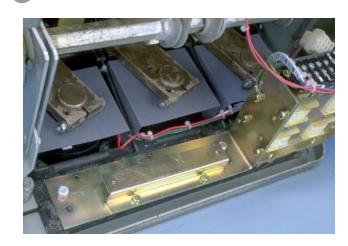
B. Mount the PT Module to the "Z" Mounting Bracket as shown, using the (2) .138-32 × .375" screws, (2) lock washers, and (2) flat washers supplied. The Glass Poly Insulation Barrier must be positioned between the PT Module and the "Z" Mounting Bracket.
