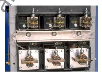
Place the CPT in front of the Breaker. Strip .250" of insulation and attach a .138" ring terminal to each wire of the CPT Harness. Connect the wires to the X1 and X2 terminals of the CPT.
