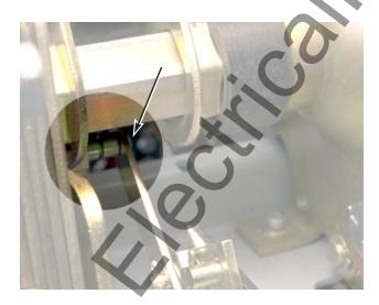
D. Align the DTA Assembly with the existing holes in the Breaker Shelf. Apply Loc-Tite® 242 to the threads then secure the DTA Assembly to the Breaker Shelf using the (2) .250-20 × .750" bolts, (2) lock washers, and (2) flat washers supplied. Note the orientation of the DTA Gap Adjustment Screw to the Trip Finger.
