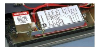
C. The PT Wires are marked for connection to Phases 1, 2, and 3 with corresponding numbers.
