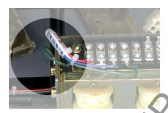
G. Secure the Sensor Harness, using the wire ties supplied, to keep it clear of any moving parts within the Breaker.
