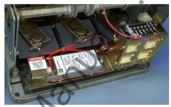
A. Align the PT Module "Z" Mounting Bracket with the holes near the bottom center of the Aux. CT Module Mounting Bracket. Secure the PT Module Mounting Bracket using the (2) .190-16 × .500" thread cutting screws, (2) lock washers, and (2) flat washers supplied.
