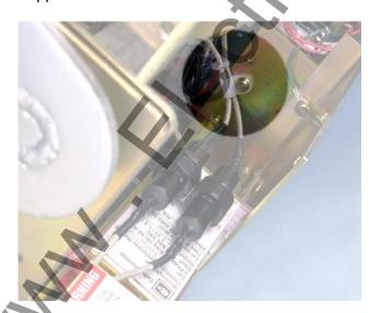
NOTE: The Line Side High Voltage Fused Wires (HV Wires) are longer than necessary and are cut during the following steps. Before cutting the wires, be sure that sufficient length is left so that the HV Wire Fuses are accessible and that the connections can be made to the correct Breaker Stabs.
