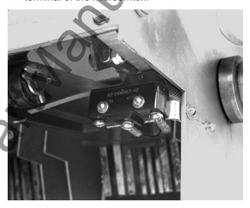
H. Use the nylon wire ties provided to dress all wiring to keep it away from any moving parts within the Breaker. Page 14 IL 33-A4H-2
