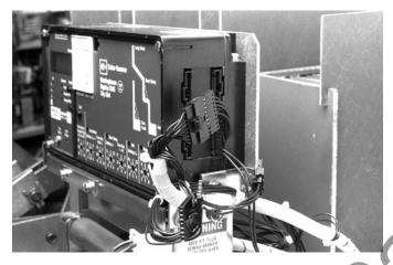
Cut the wires to length. Strip .250" of insulation and attach a .138" ring terminal to each wire. Connect the wires to the X1 and X2 terminals of the CPT.
