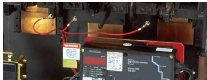
Fig. 18 PT Wires connected to the Phase Frames.
