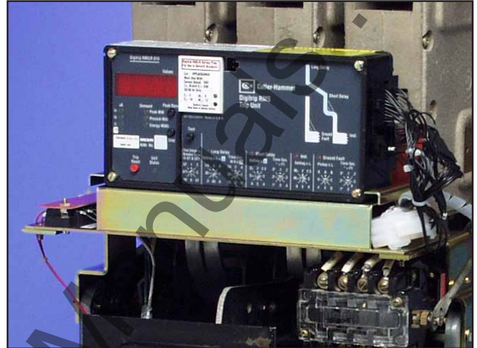
Fig. 34 Overview: Trip Unit / Aux. CT Module Assembly Installed in the Breaker
