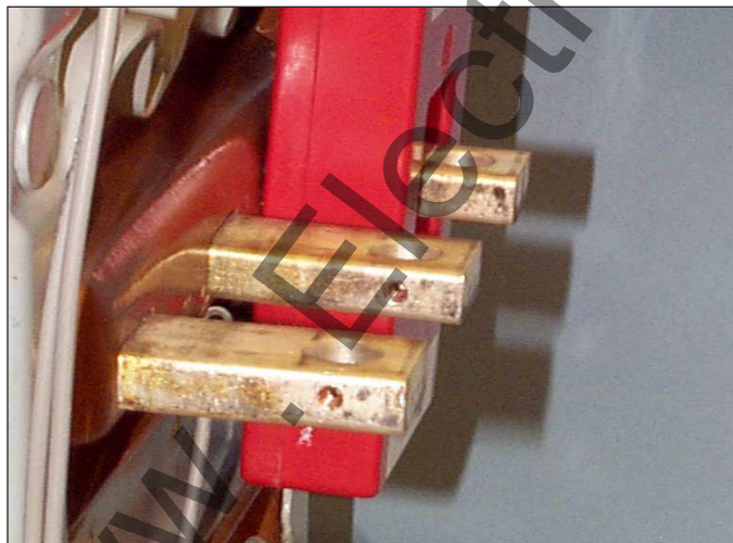
Fig. 48 Breaker Stabs Drilled and Tapped for HV Wire Connection
