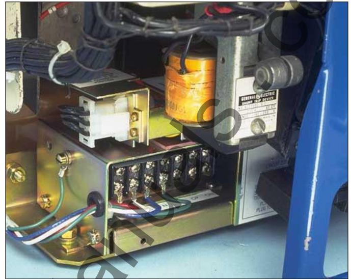
Fig. 61 Sensor Harness Connected to the Aux. CT Module
