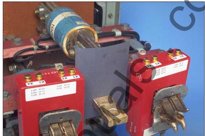
Fig. 55 Fish Paper Installed on the Phase 2 Breaker Stab
