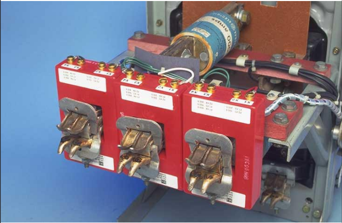
Fig. 64 Sensor Harness Connected to the Sensors
