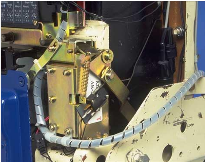
Fig. 71 External Harness Secured to the DTA Assembly
