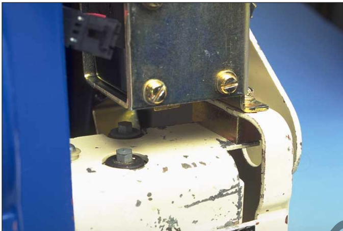
Fig. 37 PTA Assembly Mounted to the Breaker - Electrically Operated
