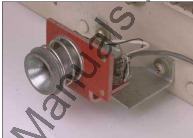
Fig. 3 Neutral CT Disconnect
