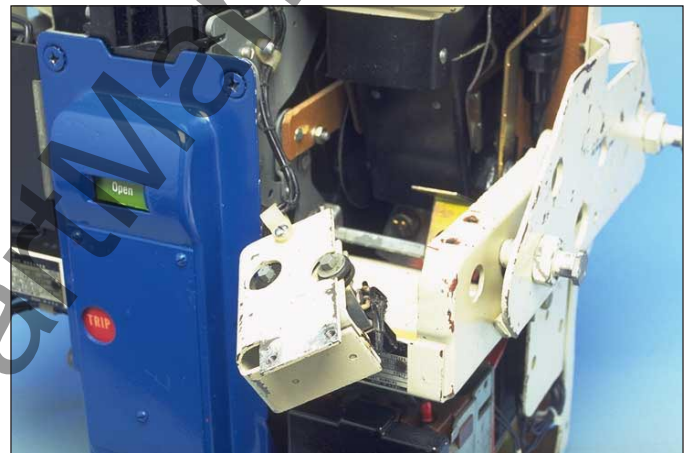
Fig. 35 Temporary Removal of the Control Relay
