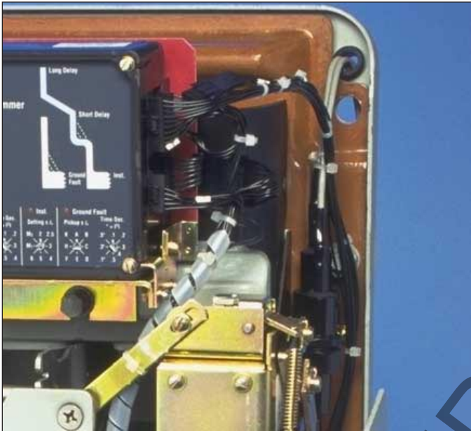
Fig. 74 CPT Harness Connected to the Trip Unit and External Harness
