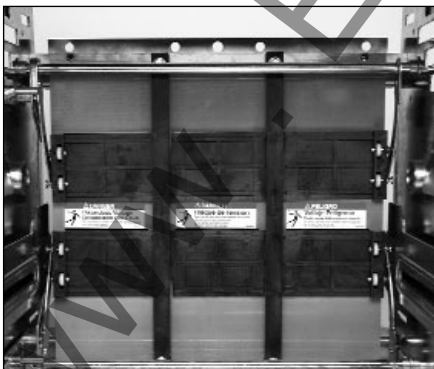
Figure 12 Safety Shutters in Closed Position
