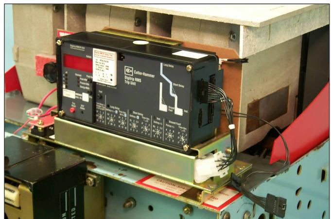
Fig. 60 Rating Plug and Aux. CT Harness Installed.
