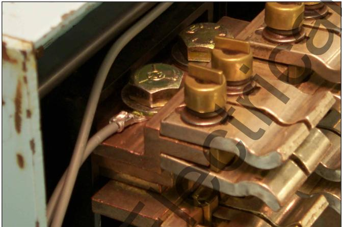
Fig. 32 HV Wires Connected to Top Secured Finger Clusters.
