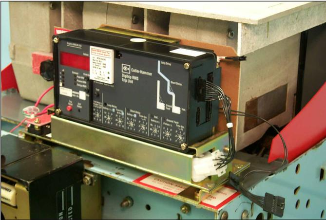
Fig. 52 Overview: Aux. CT Assembly and Trip Unit Installed on the Breaker.
