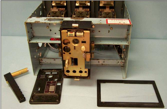
Fig. 3 Charging Handle, Face Plate, and Floating Trim Removed from the Breaker.
