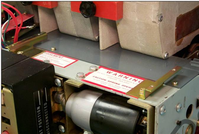
Fig. 55 Aux. CT Module Mounting Brackets Installed on the Breaker.
