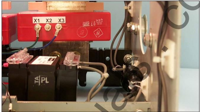
Fig. 33 HV Fuses and Wires Secured Away from Moving Breaker.
