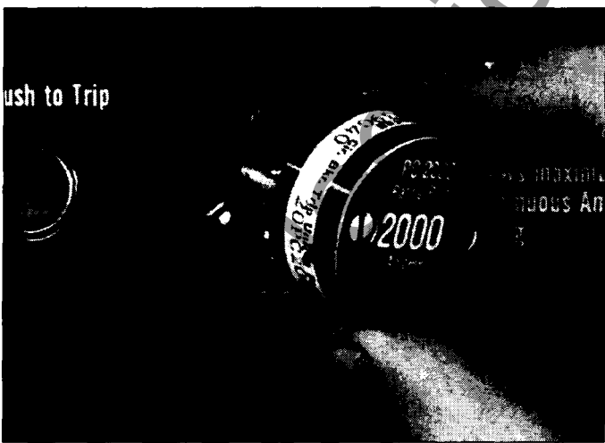
Fig. 4 Installation of PC Rating Plug
