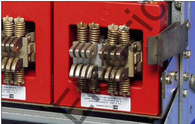
Fig. 55 Securing the Sensor Mounting Platform
