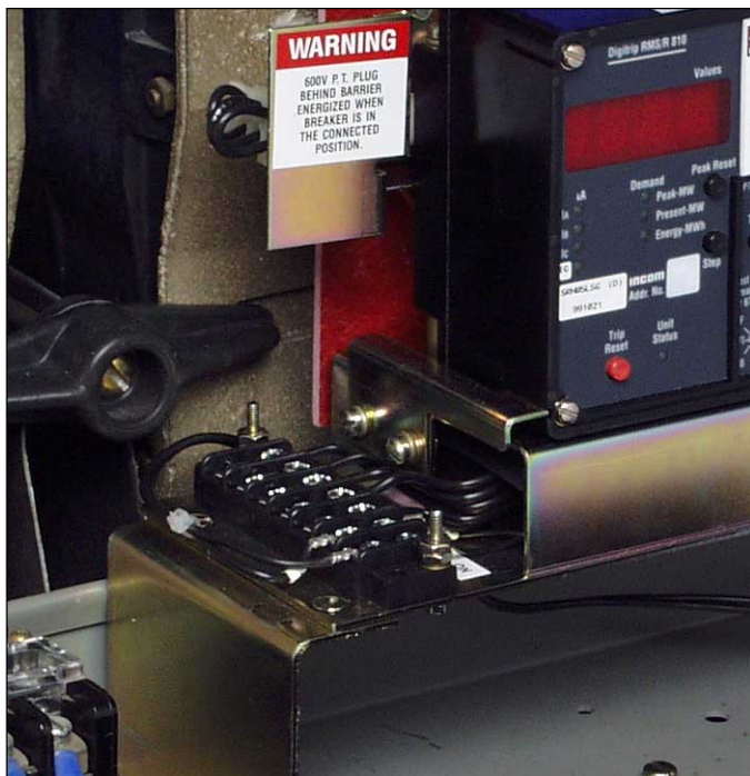
Fig. 57 Connecting the DTA Harness
