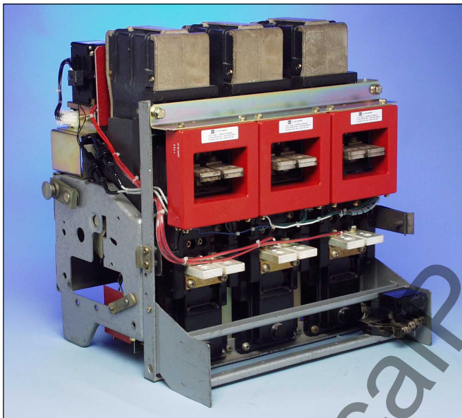
Fig. 50 Overview – Installed Top Mounted Sensors
