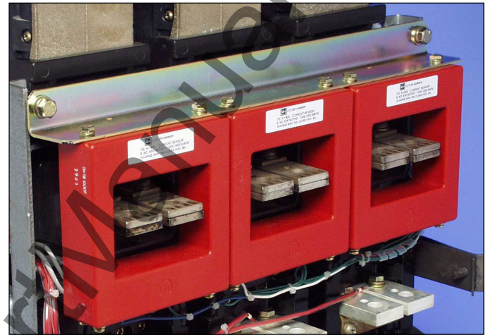
Fig. 51 Securing the Sensor Assembly to the Breaker
