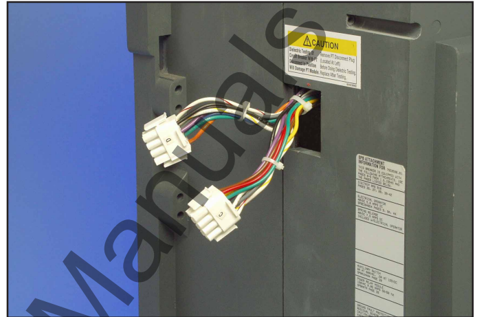
Fig. 7 Location of the C and D Blocks on Fixed Mounted, Through the Door SPB Breakers
