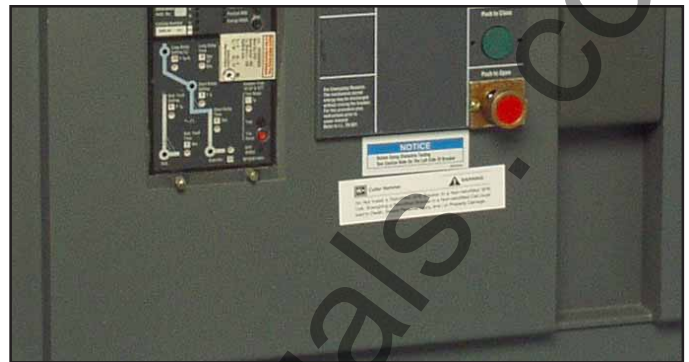
Fig. 48 SPB Warning Label Location - Large Frame Breaker
