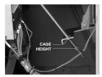
C. Connect a 24 VDC power supply to the DTA terminals; positive to positive and negative to negative. Close the Breaker manually. Energize the DTA to trip the Breaker; de-energize when the Breaker trips. Make certain that the DTA resets. If the Breaker fails to properly trip or reset, it may be necessary to readjust the cage height. Make the necessary adjustments until the trips and resets are sure and positive each time.
