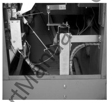
A. Using Drilling Plan "C", drill two (2) .375" diameter holes in the right Breaker Side Panel.
