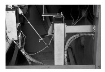
D. Route the DTA Wires from the DTA Assembly to the Aux. CT Module. Connect the "+" DTA Wire to the "OP" terminal of the Aux. CT Module and the unmarked wire to the "ON" terminal. For Kits Supplied with a PT Module Only.
