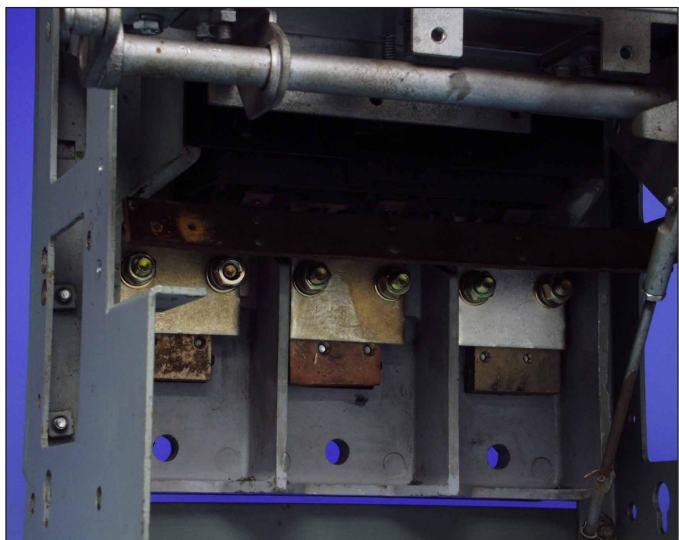
Fig. 3 Overview: Copper Connectors Installed in the Breaker
