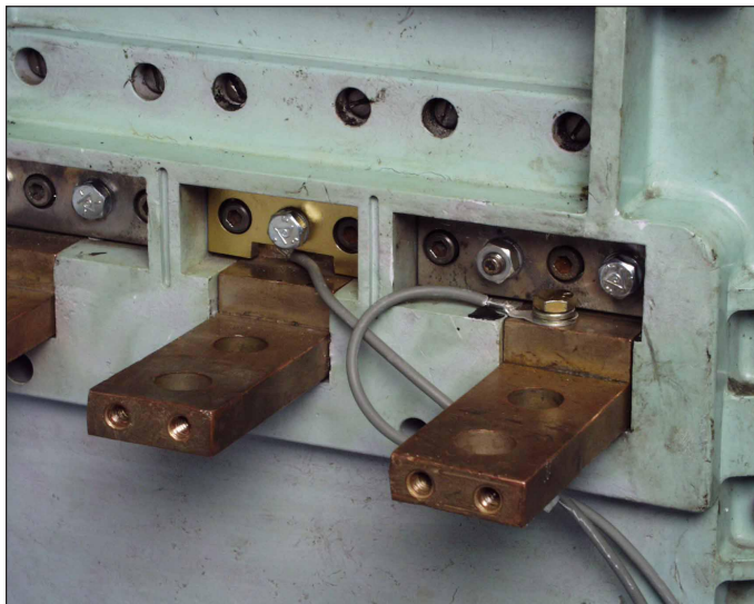
Fig. 46 New Retaining Plate Installed on Phase 2
