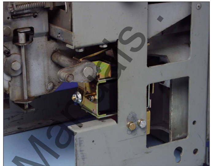
Fig. 11 Overview: DTA Installed in the Breaker
