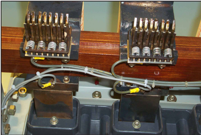
Fig. 60 HV Wires Connected to the Current Limiting Fuse Connectors.
