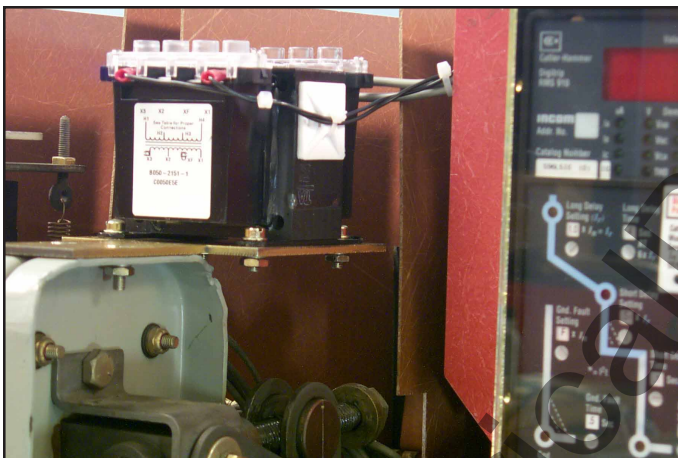
Fig. 67 Overview: All Harness and Wires Secured in the Breaker.
