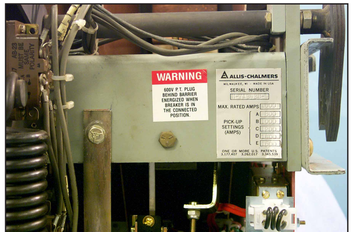
Fig. 25 PT Warning Label Installed on the Breaker.
