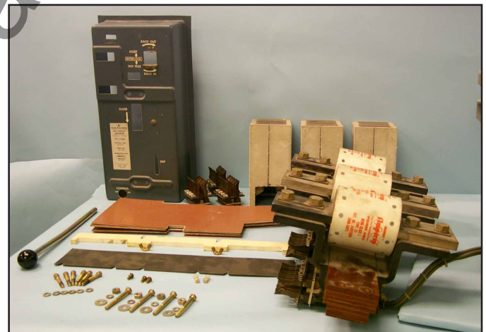
Fig. 2 Original Components Removed and Saved for Reinstallation.
