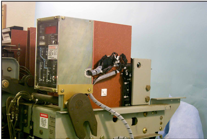
Fig. 41 Overview: External Harness Connected to the Trip Unit.
