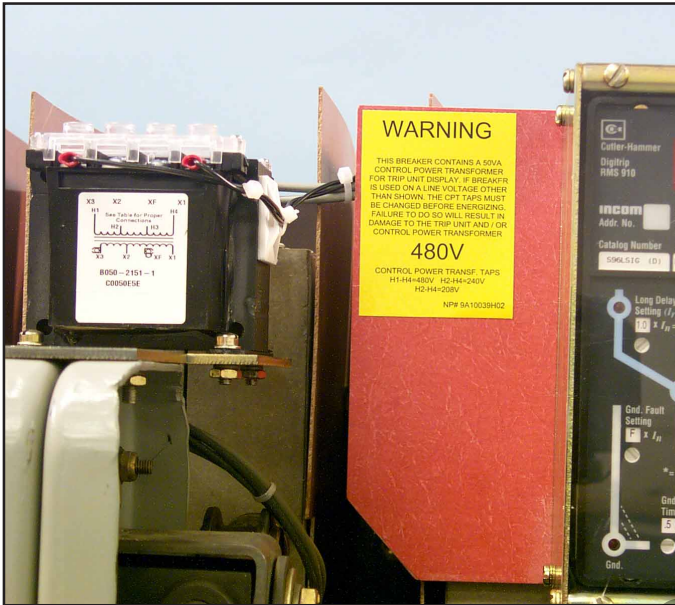
Fig. 50 Overview: CPT Module Installed on the Breaker.
