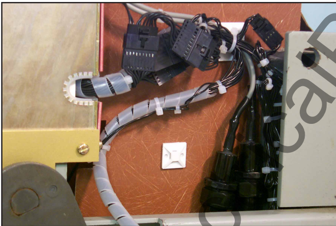
Fig. 61 HV Fuses Secured to the Breaker.
