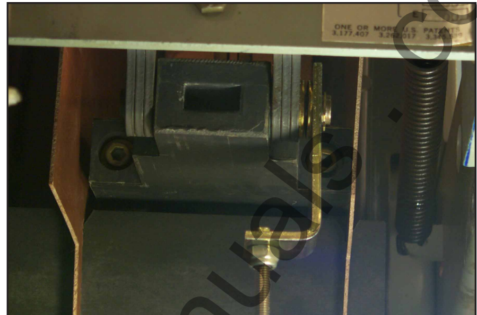
Fig. 10 Reset Link Assembly Installed on the Breaker Pole Shaft Wrist Pin.
