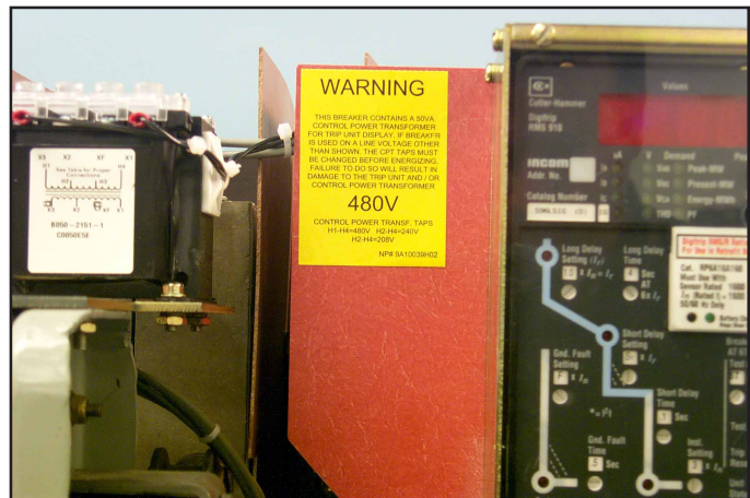
Fig. 63 CPT Voltage Label Installed on the Trip Unit Insulation Barrier.
