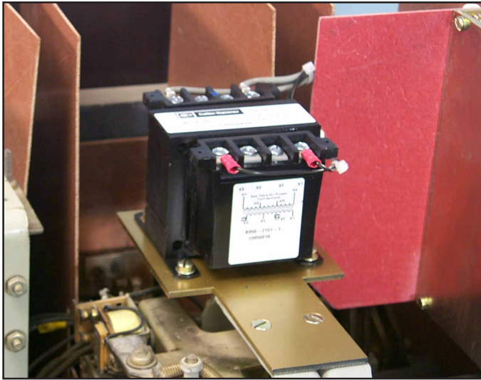
Fig. 58 Load Side HV Wires and CPT Harness Connected to the Terminals of the CPT Module.
