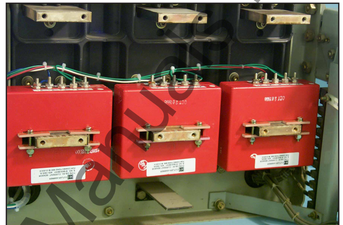
Fig. 66 Sensor Harness Connected to the Sensors.
