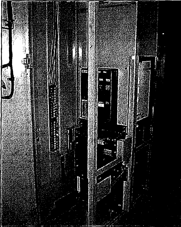
Figure 5-6 Front Racking - Position "F" (Connect)
