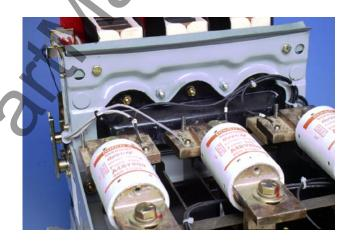
NOTE: The power convention of the Circuit Breakers is normally Top to Bottom, meaning the Top Breaker Stabs are on the Line Side of the Breaker and the Bottom Breaker Stabs are on the Load Side.
