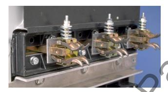
NOTE: The Line Side High Voltage Fused Wires (HV Wires) are longer than necessary and are cut during the following steps. Before cutting the wires, be sure that sufficient length is left so that the HV Wire Fuses are accessible and that the connections can be made to the correct Breaker Stabs.
