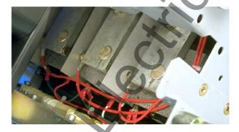
Use the nylon wire ties supplied to dress all wires to keep them away from any moving parts within the Breaker.
