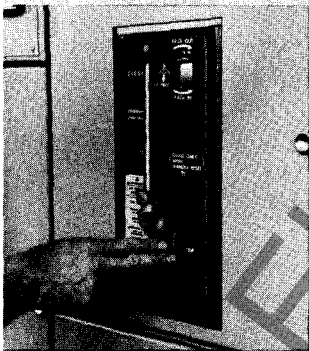
D. Depressing the interlock shutter exposes the racking screw. With the shutter depressed, the breaker is in the "trip-free" position and cannot be closed. The breaker can now be racked into or out of the compartment.
