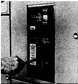
B. With the manual handle returned to vertical position, the closing lever is depressed releasing the spring energy and closing the breaker contacts.
