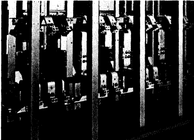
Ample space provided for incoming cables.
