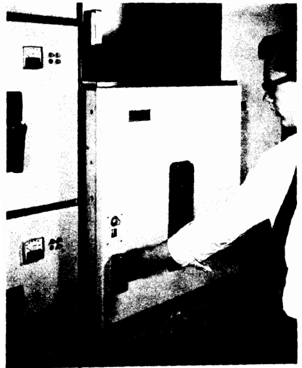
Fig. 17H (8035636) Push The Breaker In Completely And Rotate The Two Lock Links. Close The Door.
