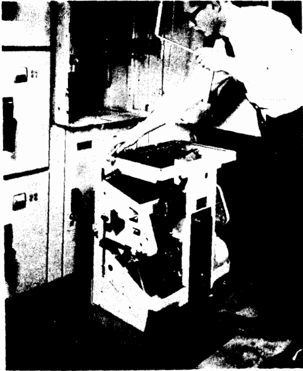
Fig. 17C (8035640) Let Out Hoist Cable. Place Hooks In Slots.
