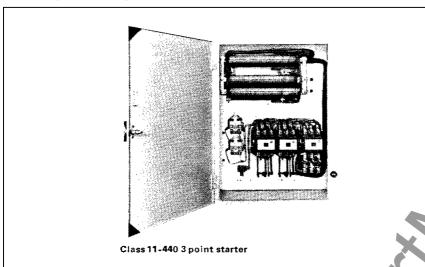
Multi-point Acceleration: These starters are designed for use on network distribution systems where the starting current limitations of the power company are such that standard across-the-line or 2-point resistance type starters will not give small enough increments of starting current.
