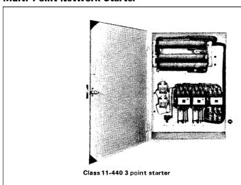
Multi-point Acceleration: These starters are designed for use on network distribution systems where the starting current limitations of the power company are such that standard across-the-line or 2-point resistance type starters will not give small enough increments of starting current.
