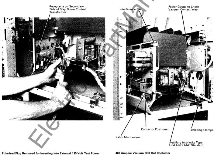
Polarized Plug Removed for Inserting into External 115 Volt Test Power Insures Against Back Feed Through Control Transformer
