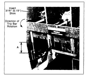
Figure 12. Operational Check of Trip Mechanism
