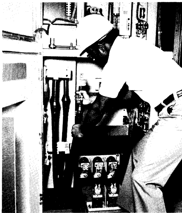
Fig. 65. Extra-width enclosure for motor cable.
