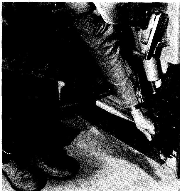
Fig. 23. Release of lintel removal catch on right end.
