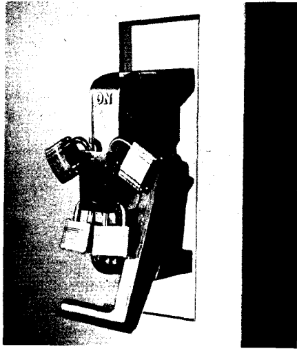
Fig. 8. Limitamp isolator handle padlocking provisions.
