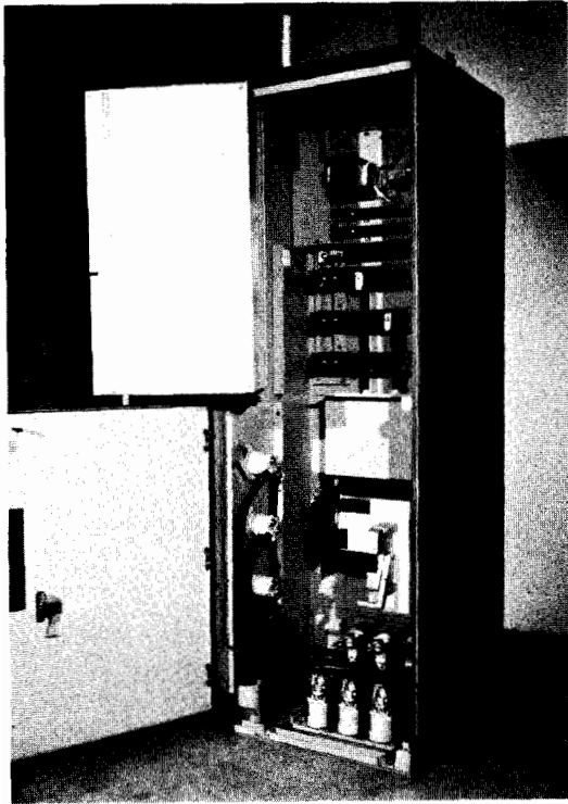
Fig. 31. One-high enclosure with contactor and barriers removed, showing left side of enclosure and terminal points on bus.
