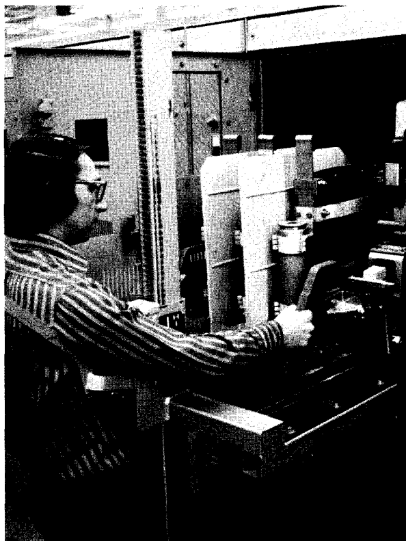
Fig. 36. Removing contactor, using Cat. No. 116C9918G1 lift.
