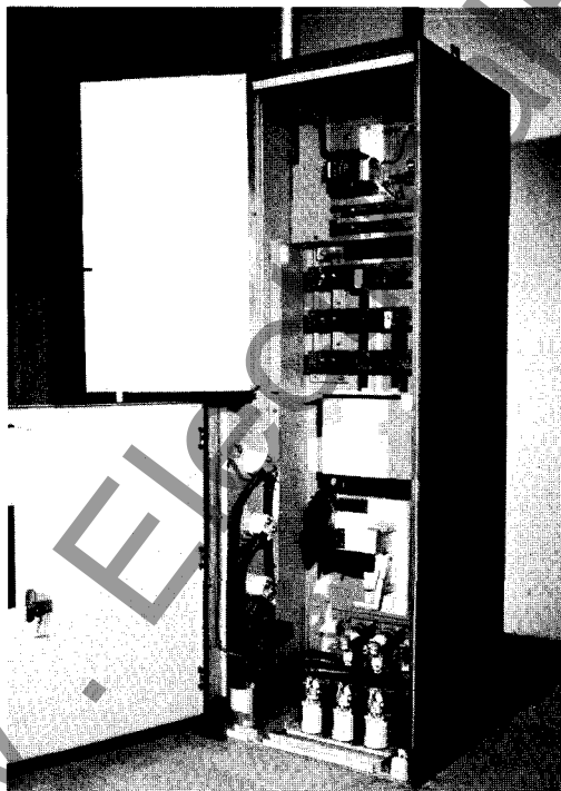
Fig. 54. One-high enclosure with contactor and barriers removed, showing left side of enclosure and terminals on bus.
