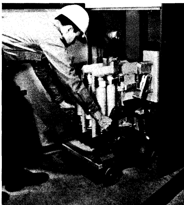
Fig. 26. Roll contactor out of enclosure.
