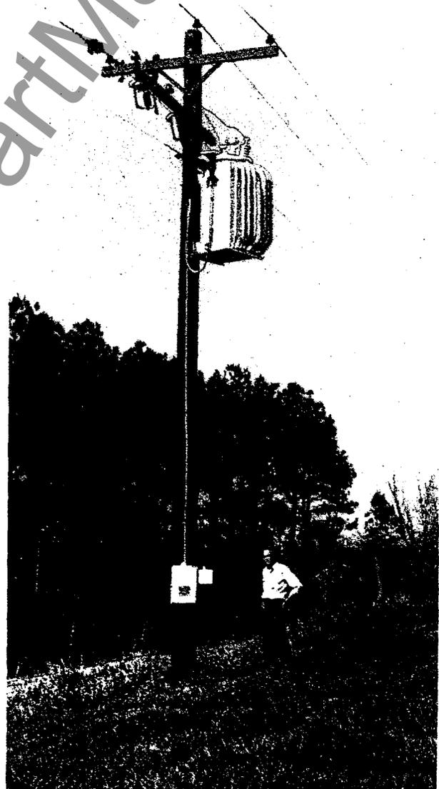
Fig. 26 Remote mounted control compartment.
