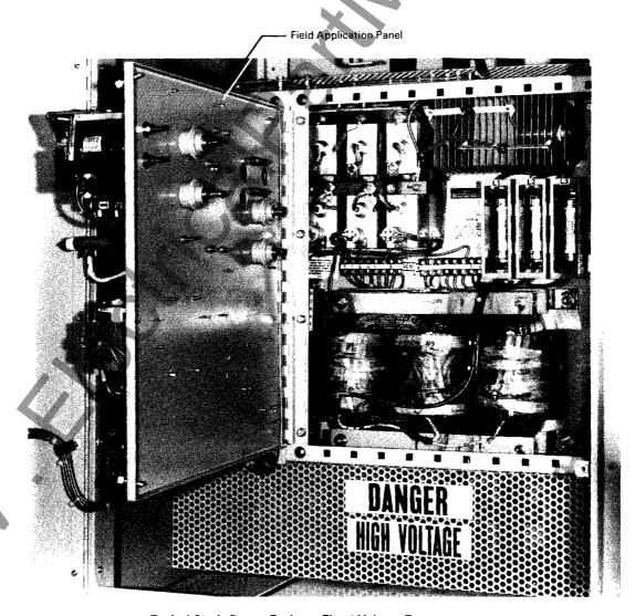
Typical Static Power Exciter – Fixed Voltage Type Mounted Behind "Swing-Out" Relay Field Application Panel
