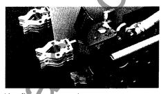
Line fingers mounted on contactor.
