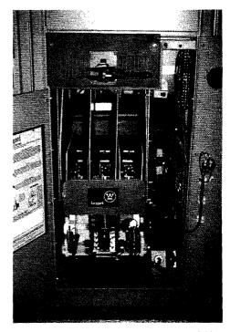
26 in. wide 50L2 air break design, with SJO Vacuum Contactor Retrofit installed. (Power fuses not installed).
