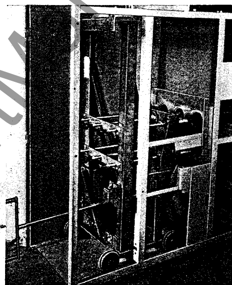
Fig. 96. Every stationary structure is checked for alignment with a master removable element.
