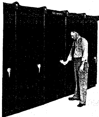
Fig. 66. Close and latch stationary structure door—breaker side.
