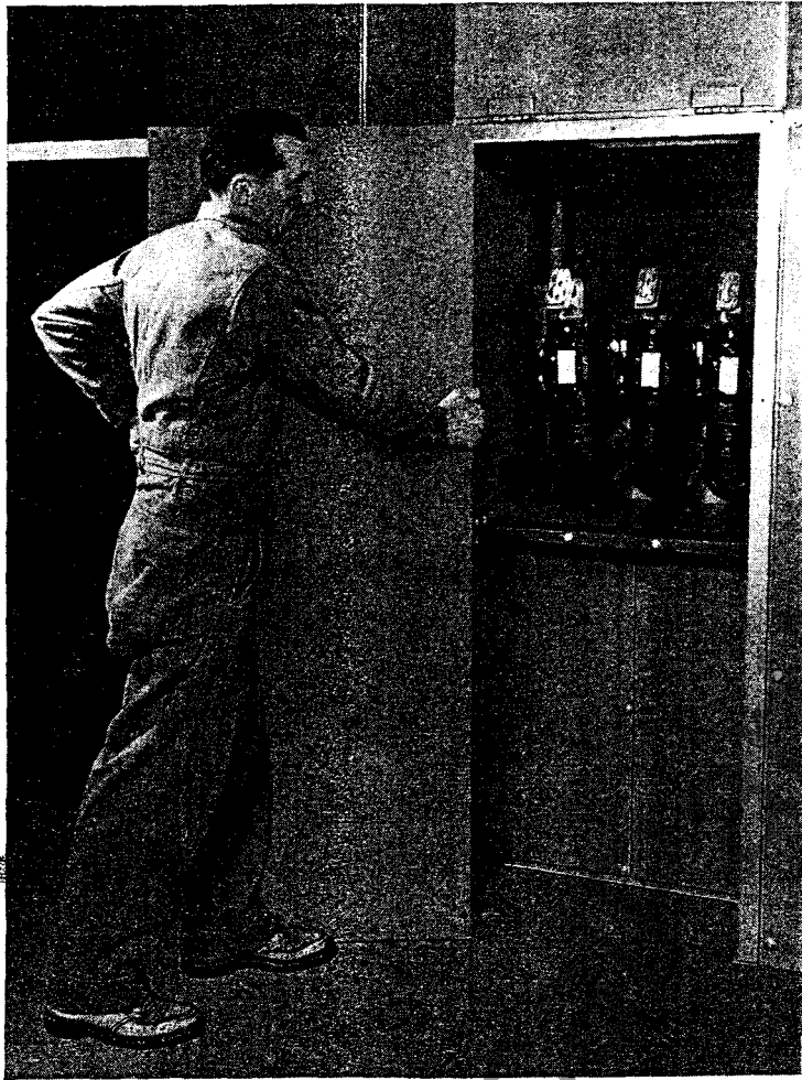
Fig. 12. Remove rear barrier for inspection of transformers and connections. Barrier is removed by unscrewing a few bolts.
