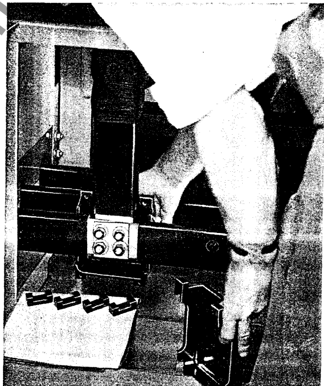
Fig. 17. Bus taps enclosed . . . Moldarta® compound box easily installed and filled with insulating compound.
