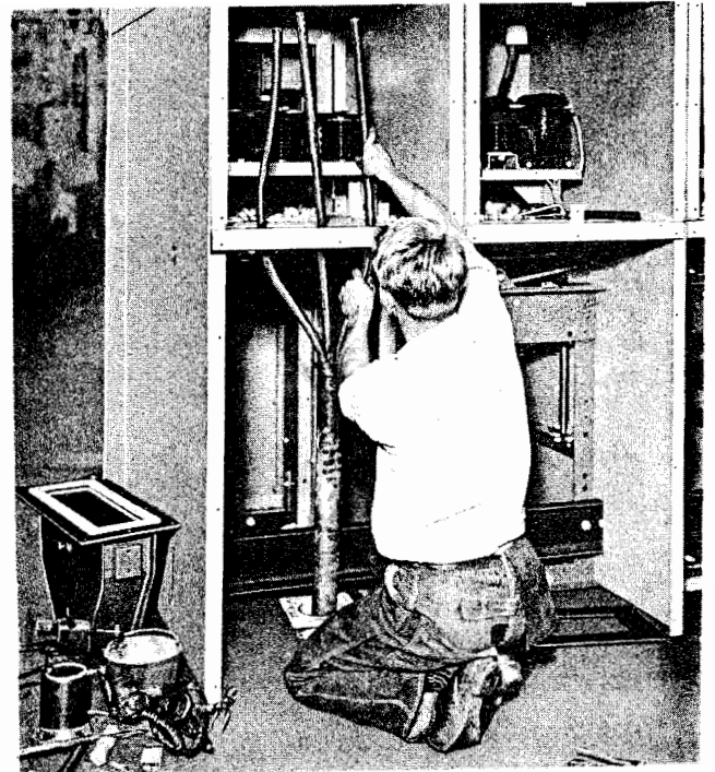
Fig. 28 Approximating Final Position
