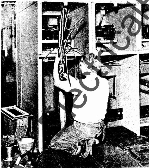
Fig. 27 Removing Belt and Interphase Insulation
