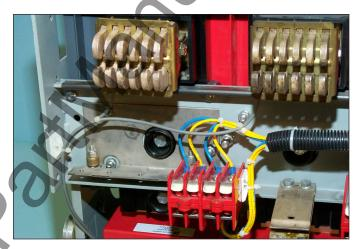
Fig. 33 HV Fuses and Wires Secured Away from Moving Breaker.
