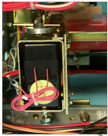
Fig. 46 DTA Mounted to the Bottom Front Breaker Channel.
