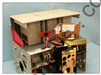
Fig. 53 Original Components Reinstalled on the Breaker.
