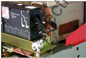
Fig. 64 External Harness Connections at the Trip Unit.
