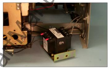
Fig. 24 HV and CPT Wires Connected to the CPT Module.
