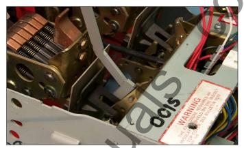
Fig. 47 Slow Close Handle Engaged in the Closing Link.
