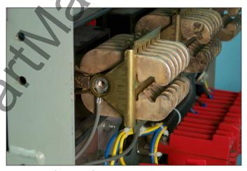
Fig. 30 Correct Orientation of the HV Wire Ring Terminals.
