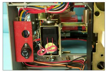
Fig. 42 Overview: DTA Installed in the Breaker.
