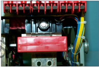
Fig. 7 Sensor and Spacers Installed on a Jumper.
