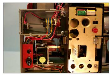
Fig. 51 Routing and Securing of the Original and New Wiring.
