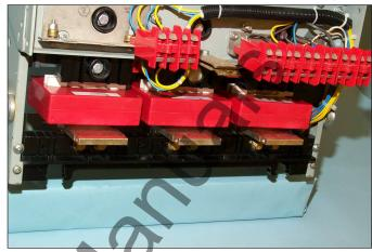
Fig. 4 Overview: Sensors Installed in the Breaker.
