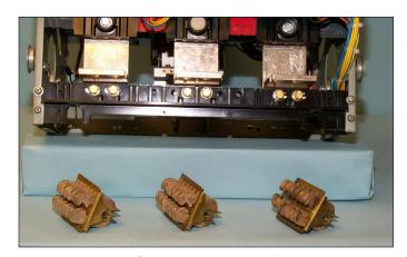
Fig. 5 Finger Clusters Removed from the Bottom Load Terminals (Electrically Operated).
