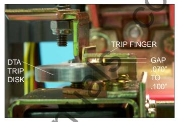
Fig. 50 Proper Air Gap Adjustment.
