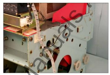
Fig. 65 External Harness Secured to the Side of the Breaker.
