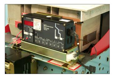
Fig. 60 Rating Plug and Aux. CT Harness Installed.
