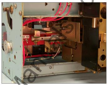
Fig. 35 Overview: Trip Finger Installed in the Breaker - Long Trip Shaft.
