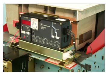
Fig. 52 Overview: Aux. CT Assembly and Trip Unit Installed on the Breaker.
