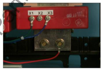
Fig. 16 PT Wires Connected to the Jumper Bolts.
