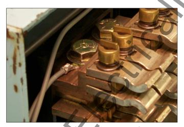
Fig. 32 HV Wires Connected to Top Secured Finger Clusters.
