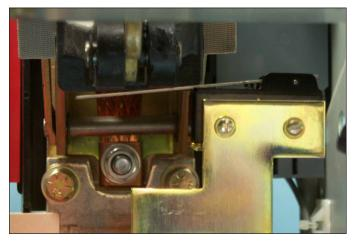
Fig. 29 Correct Engagement of the Auxiliary Switch Arm.
