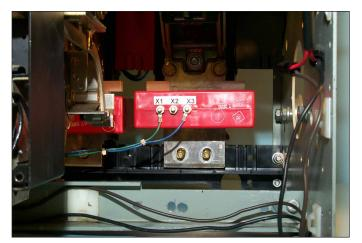
Fig. 10 Sensor Harness Connected to the Sensors.
