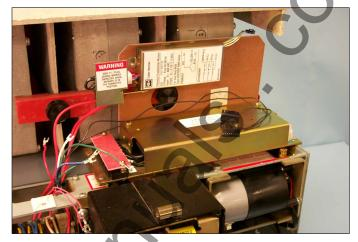
Fig. 56 Aux. CT Module Assembly Installed on the Breaker and Preliminary Routing of the Sensor Harness, DTA Wires, and CPT Wires.
