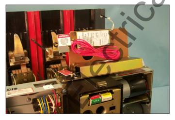
Fig. 15 Aux. CT Module Assembly Placed on the Breaker Frame.
