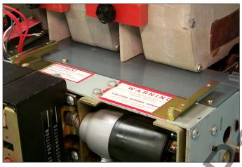
Fig. 55 Aux. CT Module Mounting Brackets Installed on the Breaker.
