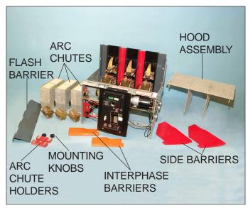
Fig. 1 Overview: Original Components Removed from the Breaker and Saved for Reinstallation.
