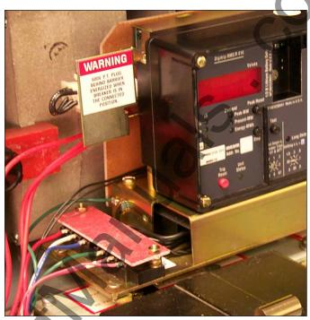
Fig. 59 Support Clips and Sensor Harness
