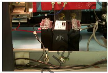
Fig. 27 CPT Assembly Installed in the Breaker.
