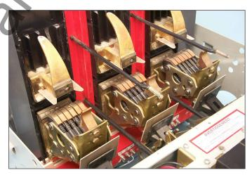
Fig. 2 Hood Assembly, Arc Chutes, Flash Barrier, Interphase Barriers, and Side Barriers Removed from the Breaker.
