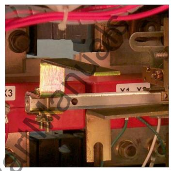
Fig. 40 Trip Finger Installed on a Long Trip Shaft.
