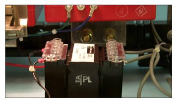
Fig. 25 Finger-Safe Covers Installed on the CPT Module.
