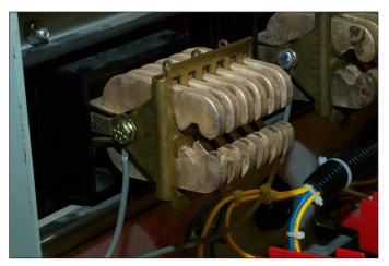
Fig. 31 HV Wires Connected to Side Secured Finger Clusters.
