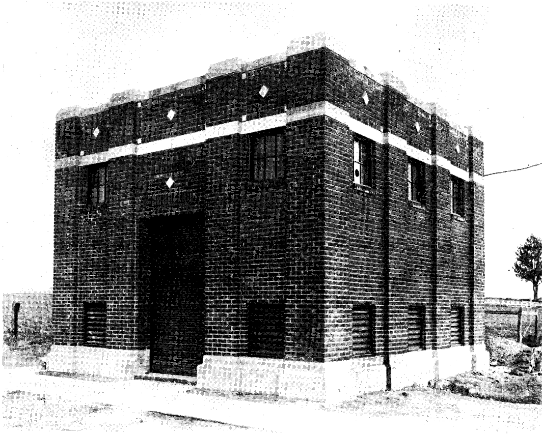
Fig. 52—Typical Automatic Substation Building for One 500 Kilowatt 600 Volt D-C. Railway Converter
