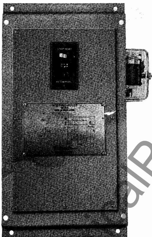
FIG. 1. Front View, TRA Relay Forced Air Cooling Control
