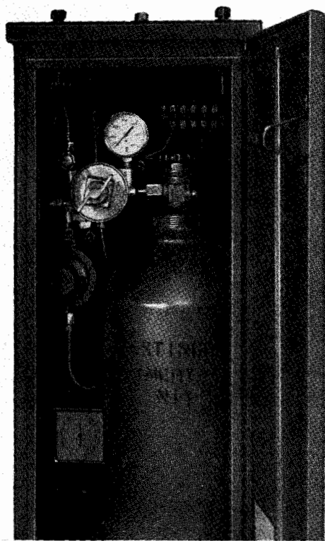
FIG. 5. Reducing Valve on Nitrogen Cylinder.
