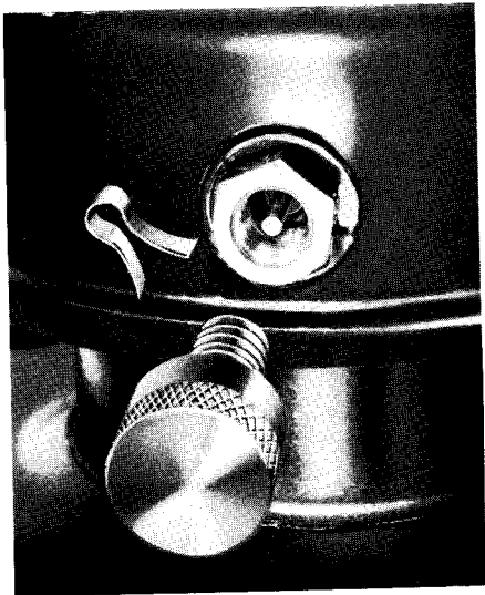
figure A: power factor test tap
