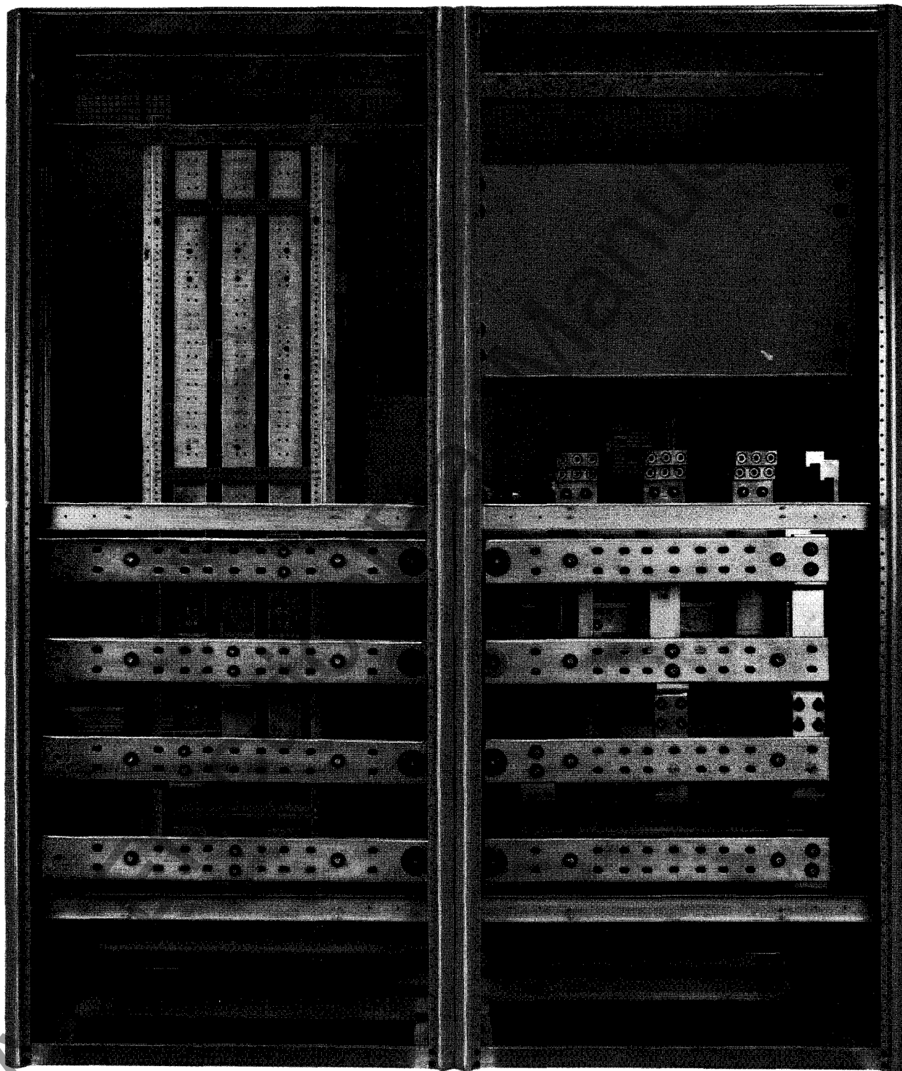
Bus Bars and Lug Construction
