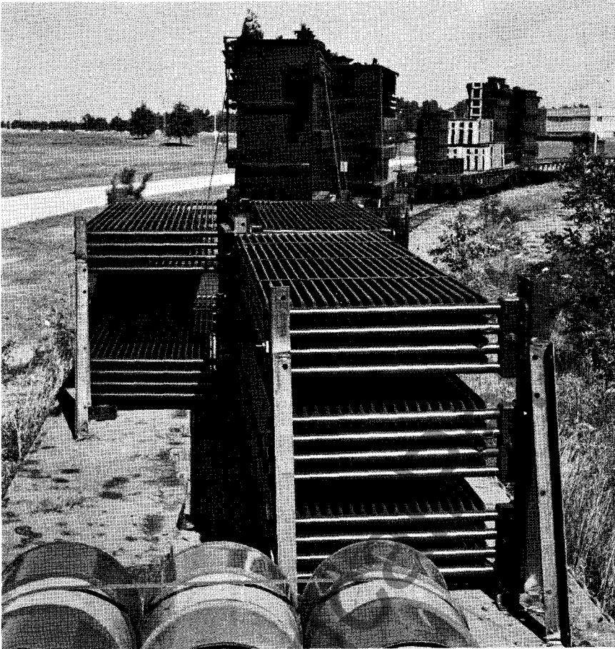
Fig. 1. Method of loading radiators for shipment
