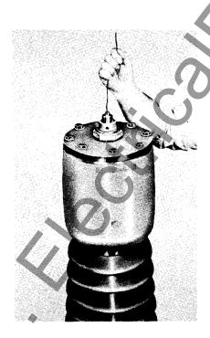
Pulling the transformer lead with attached stud up through the bushing core
