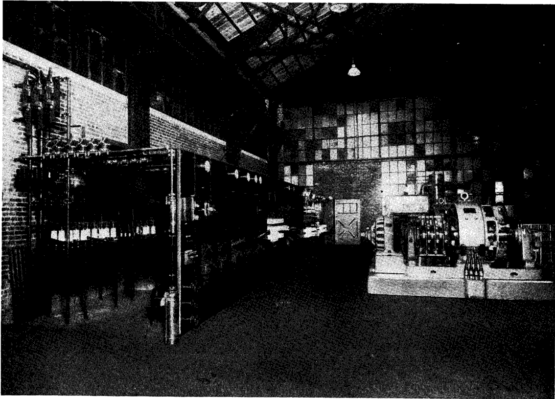
Fig. 25—Installation of Westinghouse Switchboard with Pipe Frame Structure in the Rear.
