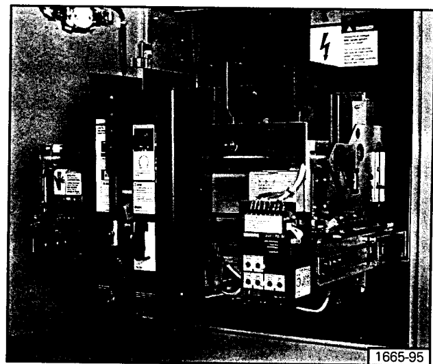
D) Continue lowering until circuit breaker rests securely on the rails. Remove the lifting yoke. The circuit breaker is now ready for inserting into the cell.
