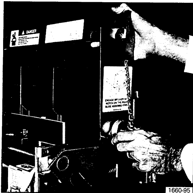
A) Attach lifting bar assembly to circuit breaker as shown above. Fasten locking screws through circuit breaker side plates and lifting plates.
