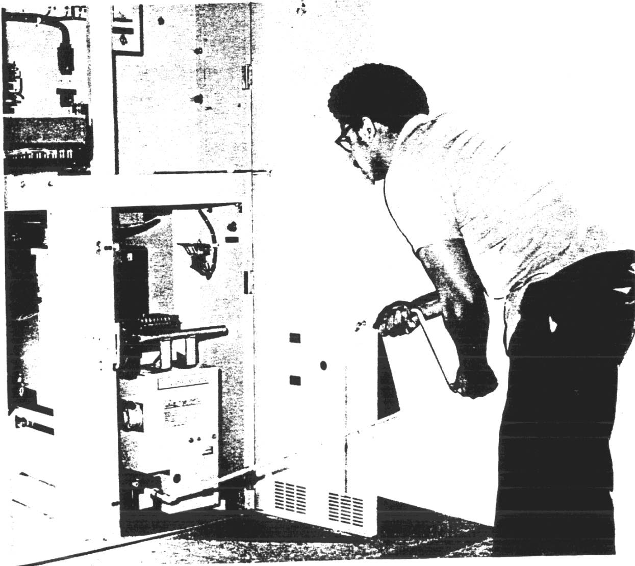
Figure 38. Breaker Racking, Manual
