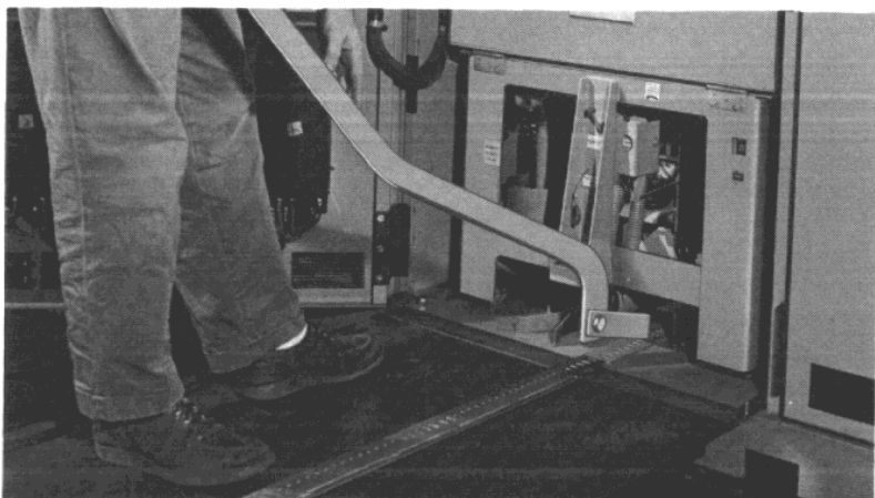
Fig. 22 — Racking of 15-kv breaker.
