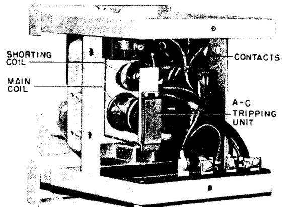
Fig. 8. (8007060) Type IAC Relay with an A-C Tripping Unit.
