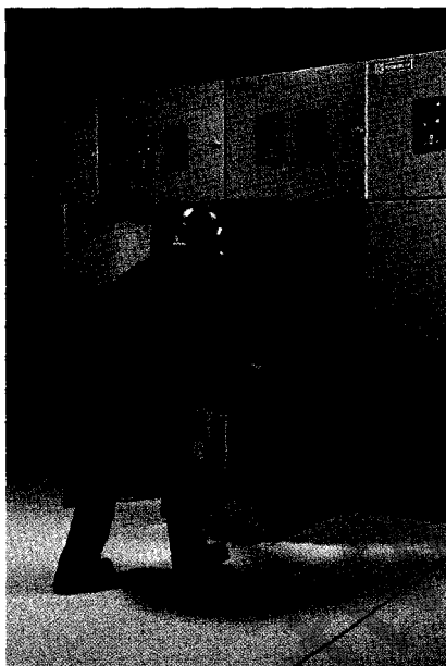
This Type DHP medium voltage switchgear line-up has been modernized with replacement panel doors (top) that include Digitrip MV Trip Units and IQ Data Plus II metering and protection devices. The operator is shown rolling a new DHP-VR Vacuum Replacement Circuit Breaker into the DHP cell.
